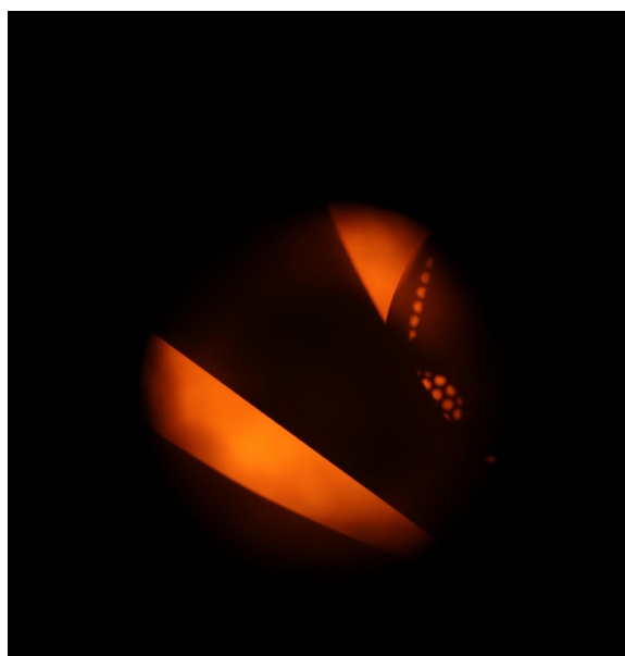
An inferno blazes in one of Princeton’s two steam boilers.
